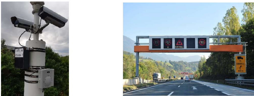
Figure 3: CCTV Camera and C-ITS Roadside Unit (left), Variable Message Sign (right)
